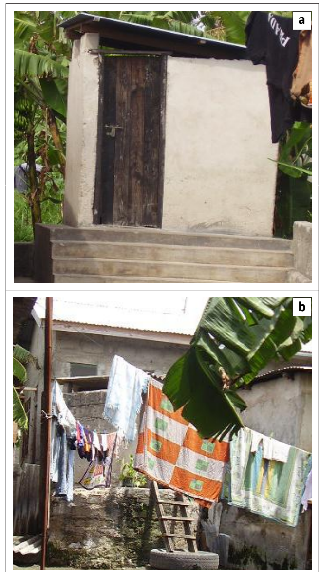
FIGURE 7: (a) Pit latrines (b) raised from plinth level.
