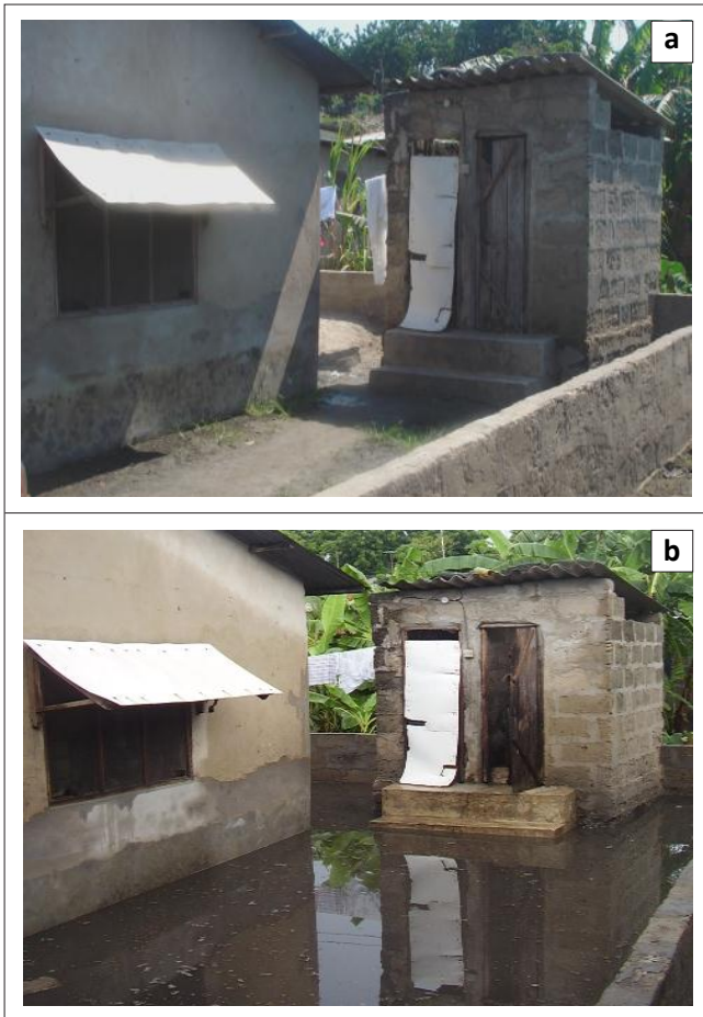
FIGURE 8: Construction of protective walls (a) before rainfall and (b) after rainfall.
