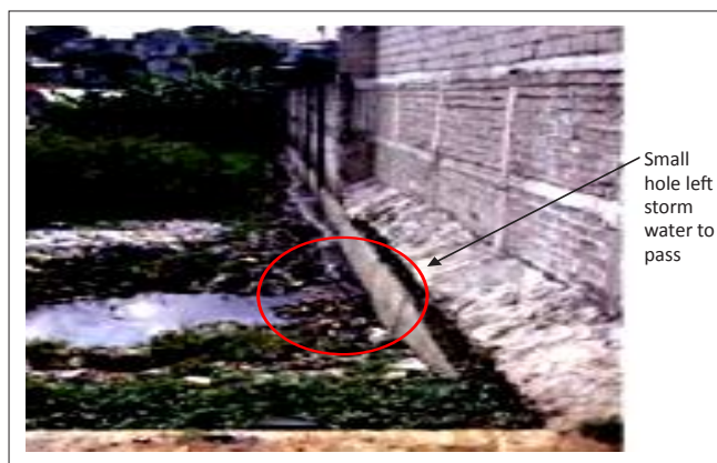
FIGURE 4: Wall constructed by Oil Com Company blocking natural water flow.
