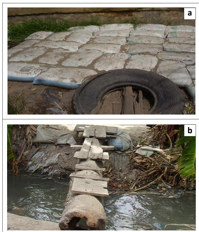
FIGURE 6: Sandbags (a) used to prevent flooding and erosion (b).
