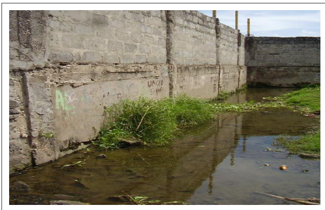
FIGURE 3: Wall constructed by Ruby Road Ways on top of the stream, blocking the natural course of the river.
