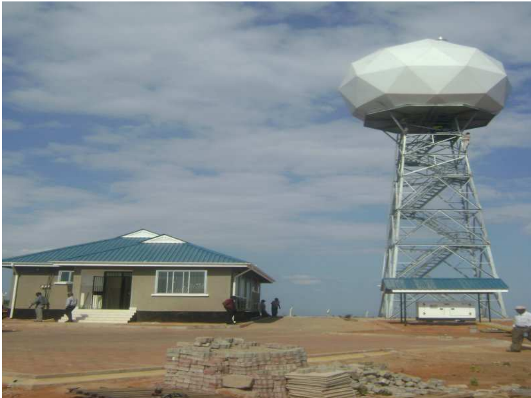
Figure 2. TMA weather radar located at Bagule, 10 km from JNIA
